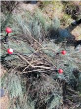
On the left: Construction of bioroll barriers. Details and construction process. Placement of escobas branch (*Cytisus* sp) at the foot of the barrier to protect the barrier support zone
